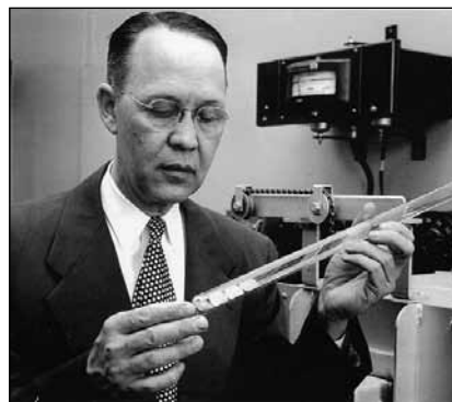
Calvin S. Fuller is shown diffusing boron into silicon to create the world’s first practical solar cell.
